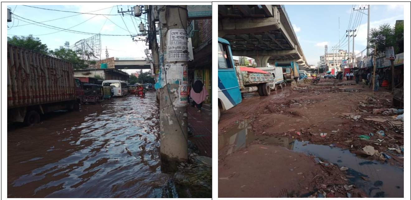
Photo: Untreated RMG chemical contaminated water flooding research locales in Ashulia
